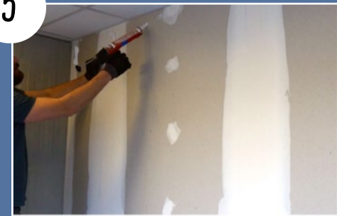
6 APPLY GLUE ON THE WALL (OR ON THE PANEL)
